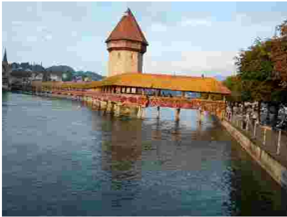
The famous wooden bridge in Lucerne
